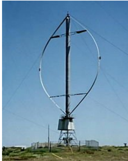
Gambar 5. Turbin angin sumbu vertical (Turbin angin Darrieus)
