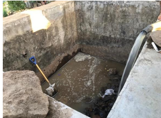
Gambar 4. Proses Pembersihan Bak Filter Air
